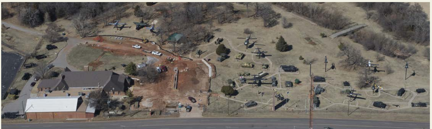
45th Infantry Division Museum parking lot renovation project
